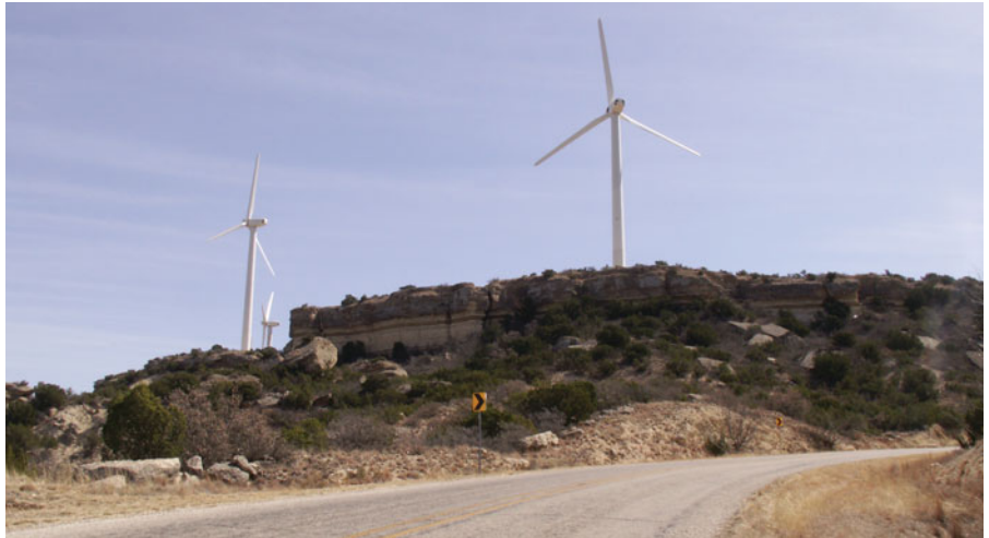
Sitting atop a ridge near the town of Fluvanna, these 230-foot-tall wind turbines are an impressive sight. The blades are 88 feet long, and the entire unit weighs 167 tons.
