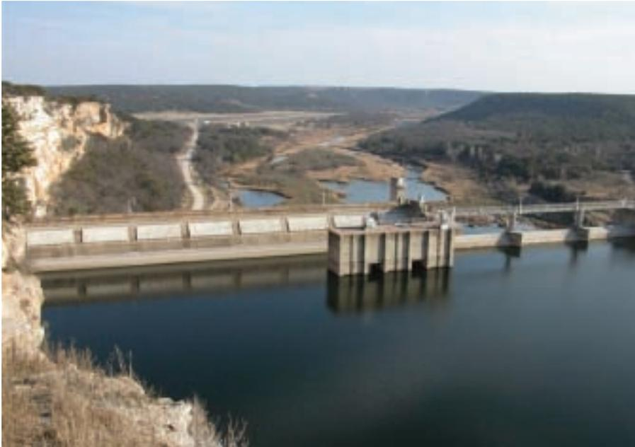
**Possum Kingdom Dam is equipped with two 12,000 kilowatt hydroelectric generating units.**
