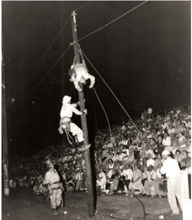
At the 1959 Annual Meeting of the Membership held at the Comanche Indian Stadium, a lineman crew demonstrates to the members how a pole-top rescue is performed.
