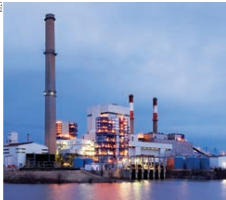
Proposed climate change actions could shut down the 37 percent of the U.S. generation capacity that comes from coal-fired plants.
